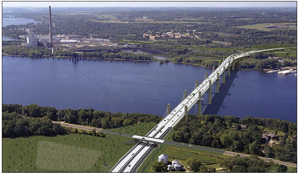
Photo simulation of the proposed river crossing looking west at the King Plant. Photo simulation from the Minnesota Department of Transportation.
