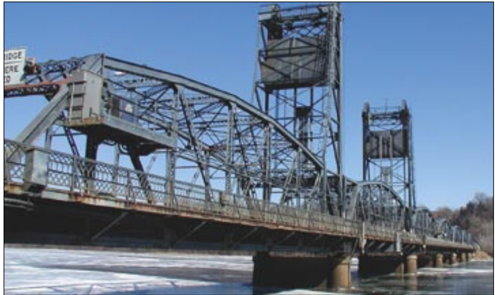
The Lift Bridge connecting St. Joseph, Wisconsin in St. Croix County with Stillwater, Minnesota was built in 1931. Traffic congestion, safety problems, and delays caused by the operation of the lift mechanism have spurred the discussion of a new river crossing. The estimated (congestion free) vehicle capacity of the Lift Bridge is 11,200 vehicles a day. A 2002 traffic study estimated 16,300 vehicles a day cross the bridge and this volume can exceed 19,000 on a summer weekend.
