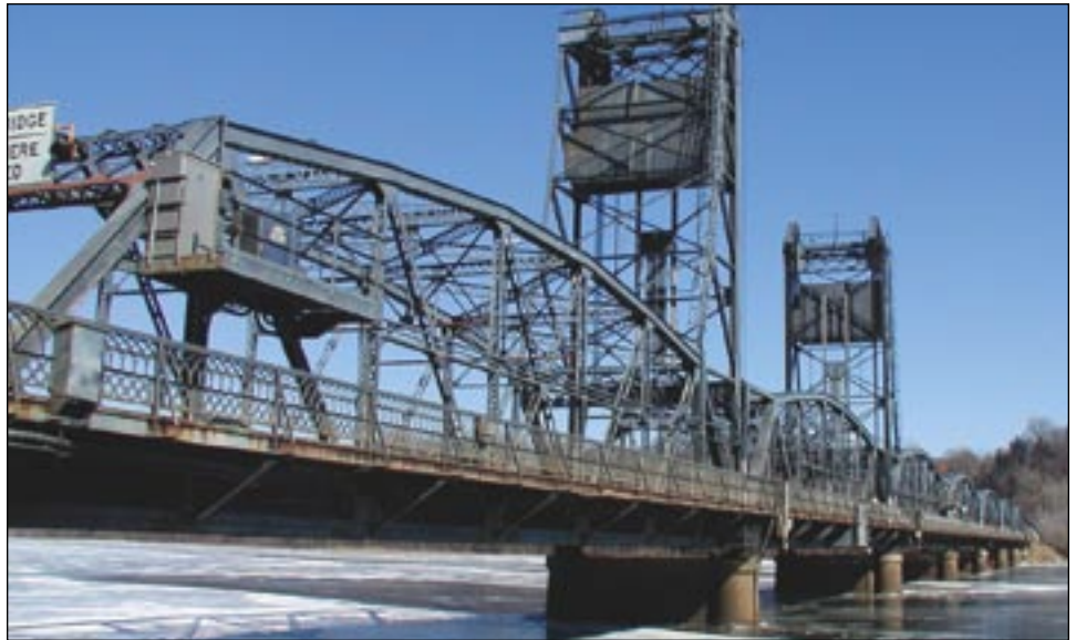
The Lift Bridge connecting St. Joseph, Wisconsin in St. Croix County with Stillwater, Minnesota was built in 1931. Traffic congestion, safety problems, and delays caused by the operation of the lift mechanism have spurred the discussion of a new river crossing. The estimated (congestion free) vehicle capacity of the Lift Bridge is 11,200 vehicles a day. A 2002 traffic study estimated 16,300 vehicles a day cross the bridge and this volume can exceed 19,000 on a summer weekend.
