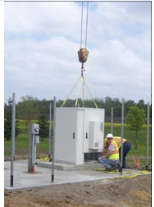
(below) Workers install the main electronics cabinet for the broadband system near the Troy Town Hall. Photos courtesy of Baldwin Telecom, Inc.
